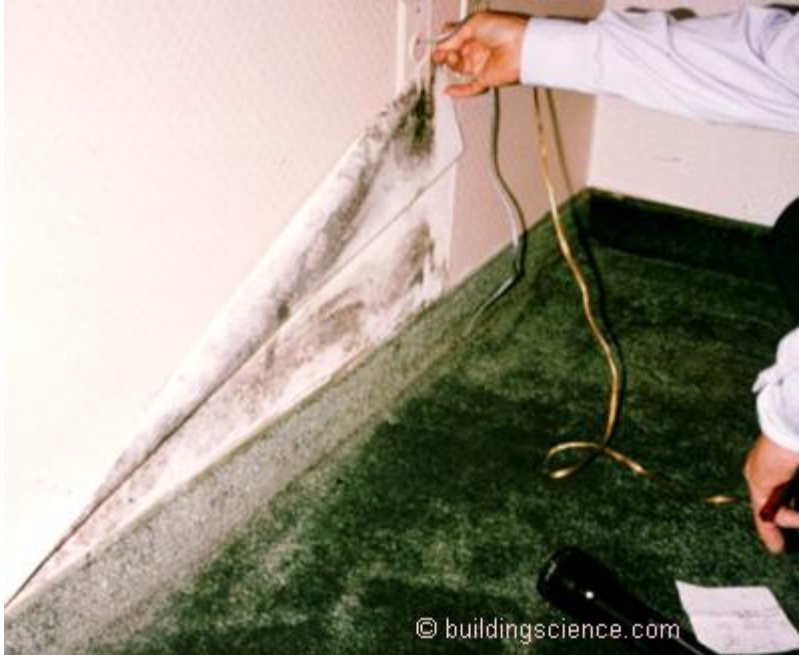
Photograph 8: Hotel Mold —Vinyl wall coverings are low perm materials that retard inward vapor movement and lead to mold growth.
