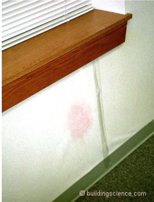
Photograph 7: Vinyl Wall Coverings and Hotels—Marriott measles, the Radisson rash, and the Hyatt hives.
