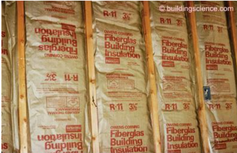
Photograph 11: Kraft-Faced Batts —Bless old timers and common sense—the kraft facing breathes during the summer allowing inward drying—polyethylene vapor barriers do not.
