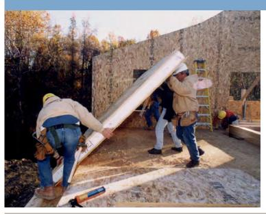
The basic design concept for SIPs is elegant in its simplicity, and offers several advantages for constructing walls and roofs. There is general agreement that SIPs provide better overall air tightness and practical thermal performance than conventionally framed walls.
